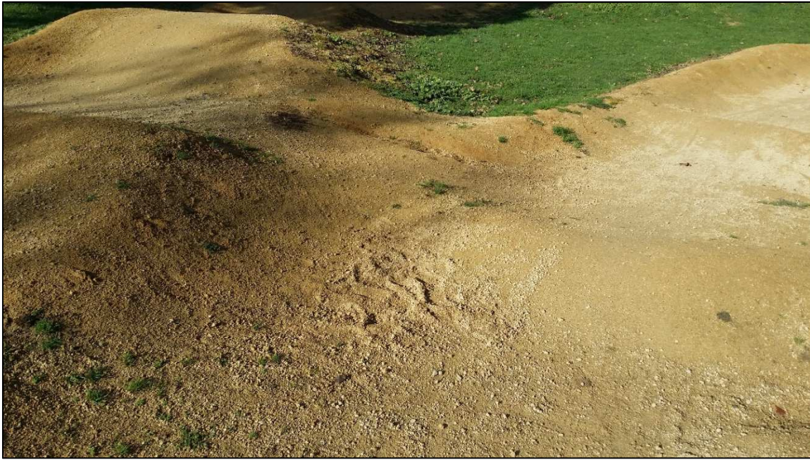
Figure 6.1: Signs of slight track deterioration, Terrace End School, Palmerston North
